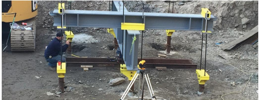
**PILES INCREASED FROM 1.5 DRILLED SHAFT CASE PILES PER DAY TO UP TO 8-9 STELCOR MICROPILES PER DAY**
