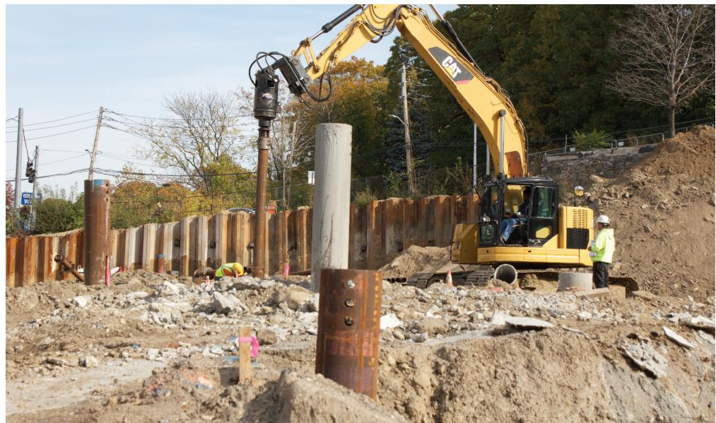
**8.625" HELICAL PIPE PILES GREATLY IMPROVED PRODUCTION TIME, RESULTING IN SIGNIFICANT COST SAVINGS**
