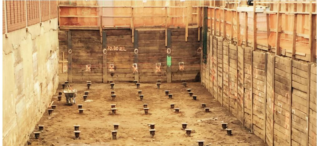
**STELCOR WAS TESTED TO 40 TONS (31 TONS WAS REQUIRED). THE PILE COUNT WAS REDUCED BY 36%**
