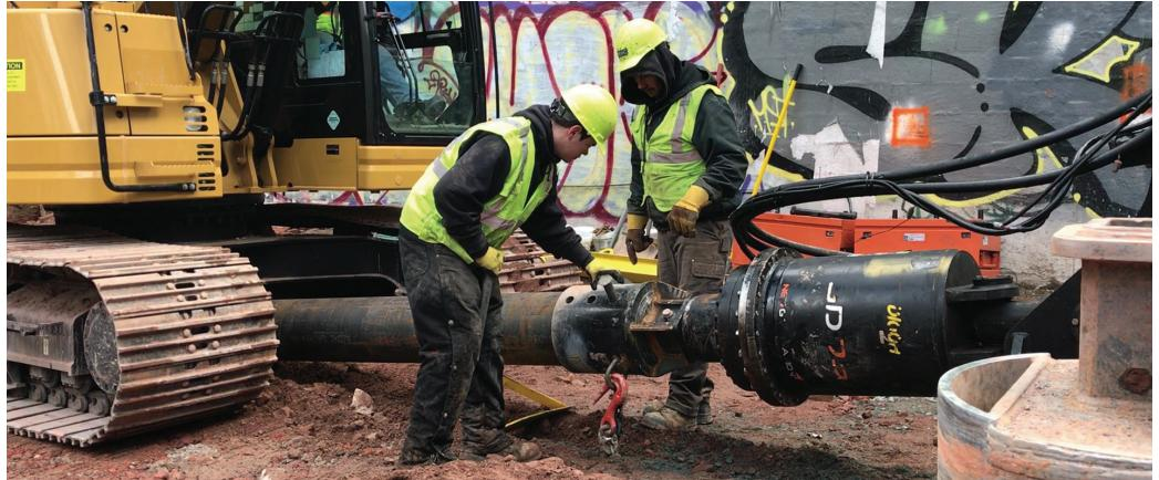
**DESPITE HAVING TO PRE-DRILL THROUGH A GRANITE LAYER AT MANY PILE LOCATIONS, HELICAL PIPE PILES REMAINED THE MOST COST EFFECTIVE PILING METHOD FOR THIS SITE.**
