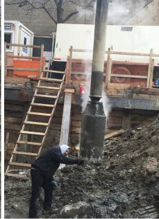
PILES INCREASED FROM 1.5 DRILLED SHAFT CASE PILES PER DAY TO UP TO 8-9 STELCOR MICROPILES PER DAY
